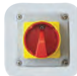
Electrical isolator Fitted to fan for security (optional)
